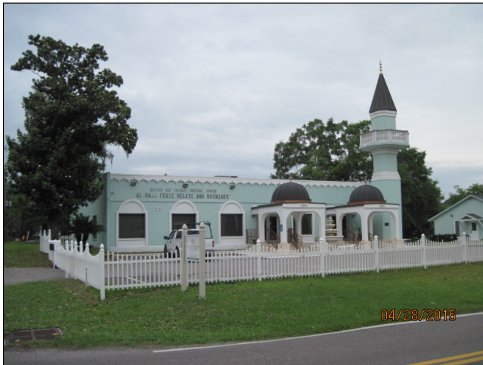
Mosque facility, 2131 Art Museum Drive
