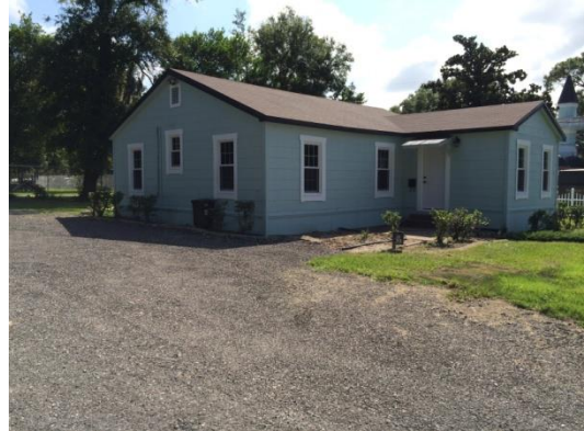
Building 6 - Law Office Entry
