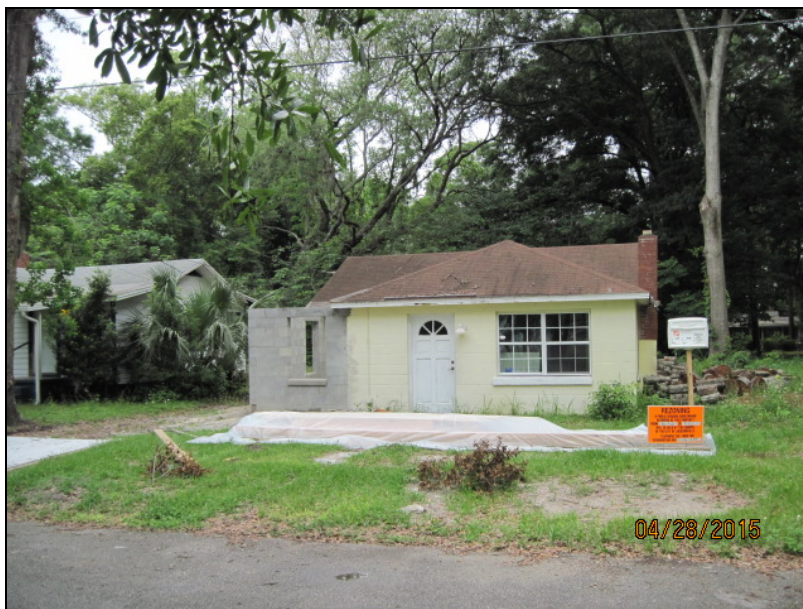
Single-family home for clergy, 4723 Pinedale Avenue
